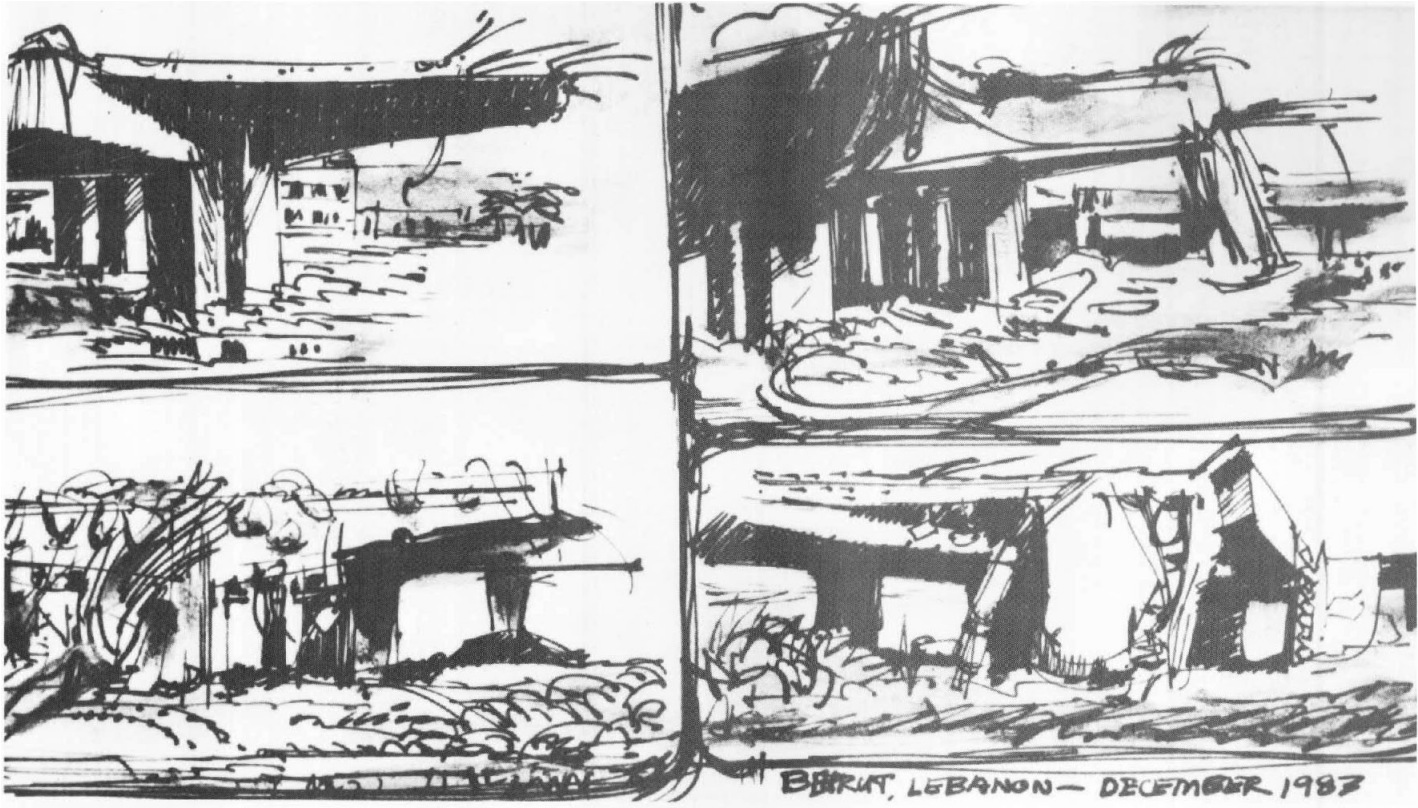
Above, these four perspectives of the former BLT headquarters ruins emphasize the destructive force of the explosion that left rods reinforcing the concrete bent and exposed.
